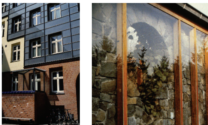
Figure 43: Indirect solar gains The walls absorb and store solar heat. Left: Renovated dwellings in Copenhagen. Dark painted plaster behind transparent insulation covered by glass. Right: Stone wall behind a layer of glass.
