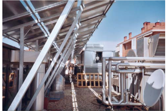
Figure 12: Solar collectors and DEC unit mounted on the roof at Mataró Library (source: Aguasol)
