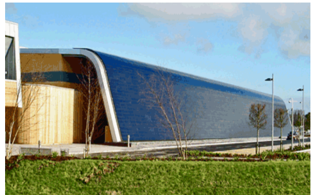
Figure 1 - The Solar Wall at the Welsh Development Agency "Technium" in St. Asaph, North Wales
