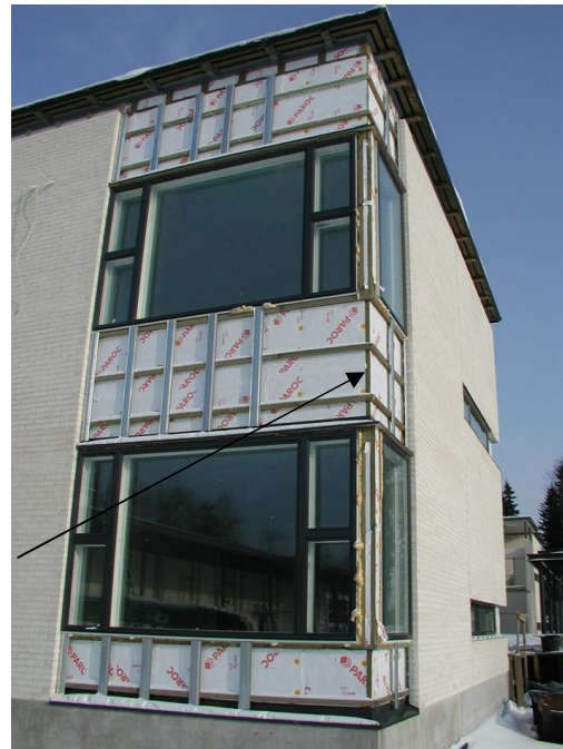
Figure 5. Window structure of the pilot building (during construction).
